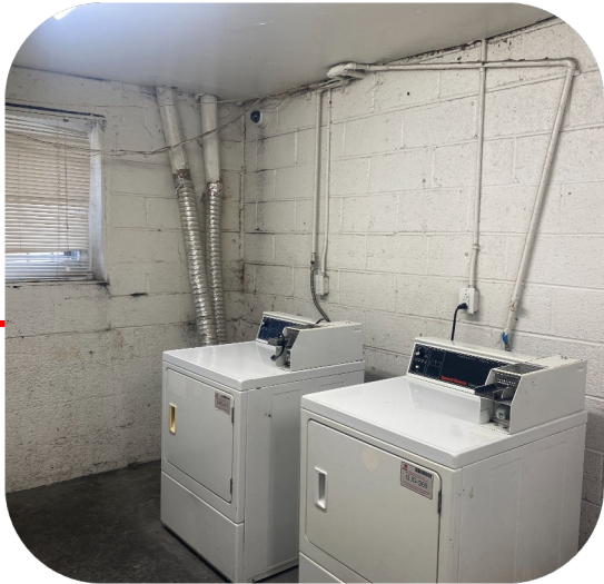
Existing vented gas dryers
