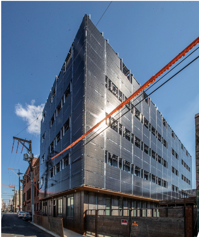
Front Flats, 174 kW array, Phila, Onion Flats
